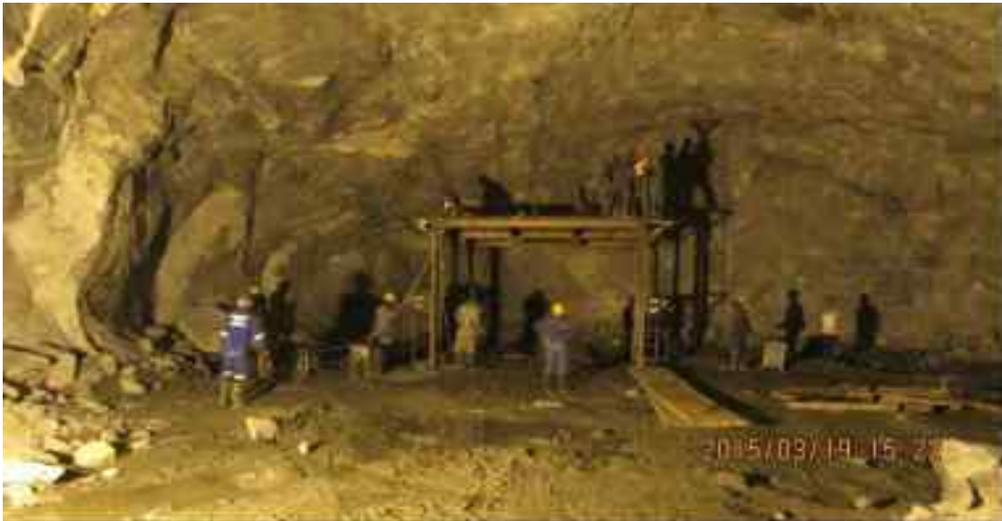
Power House Excavations
