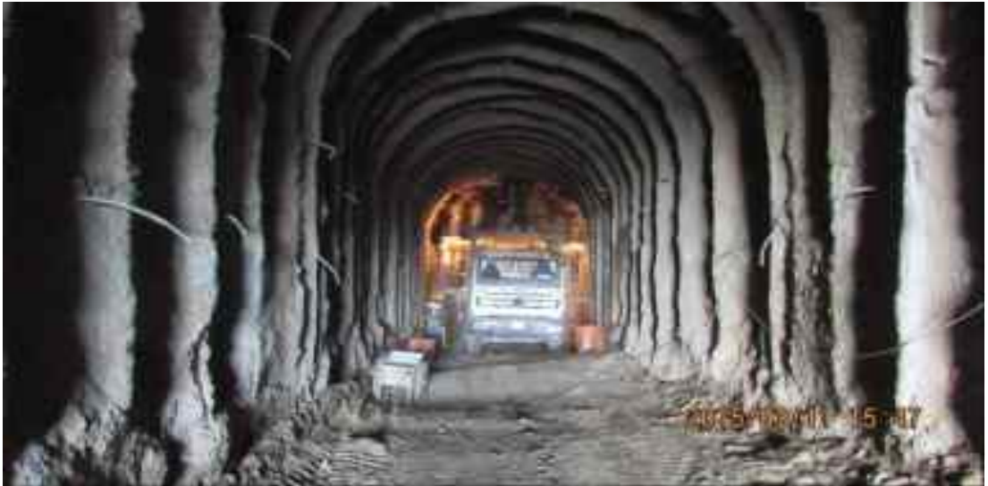
Adit 6 Excavation works
